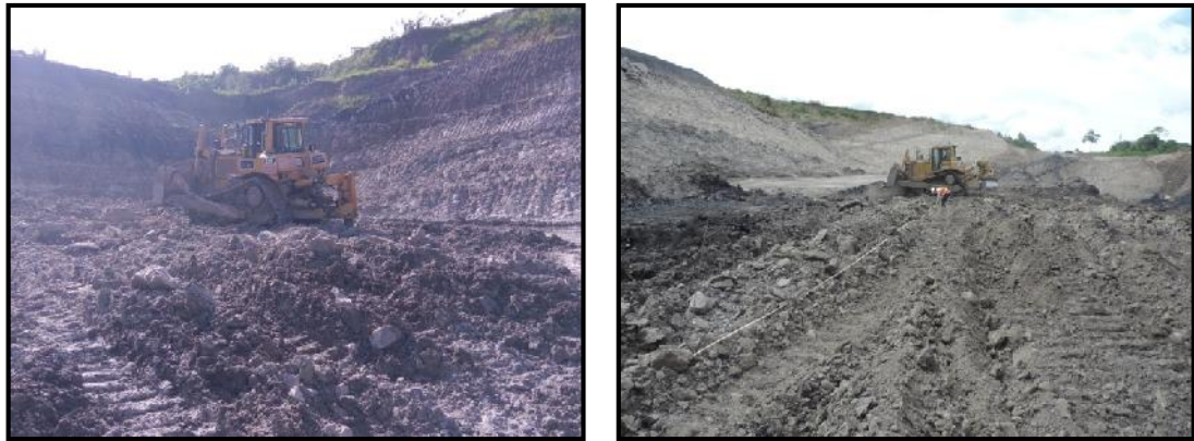
Fig 1. Ripper in the Sandstone and Siltone
