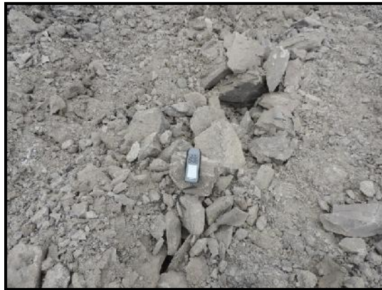
Fig 2. The result boulder of rock from the ripper Caterpillar D8R
